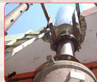
Ushma Shoshak Unit Mounted on Boiler
